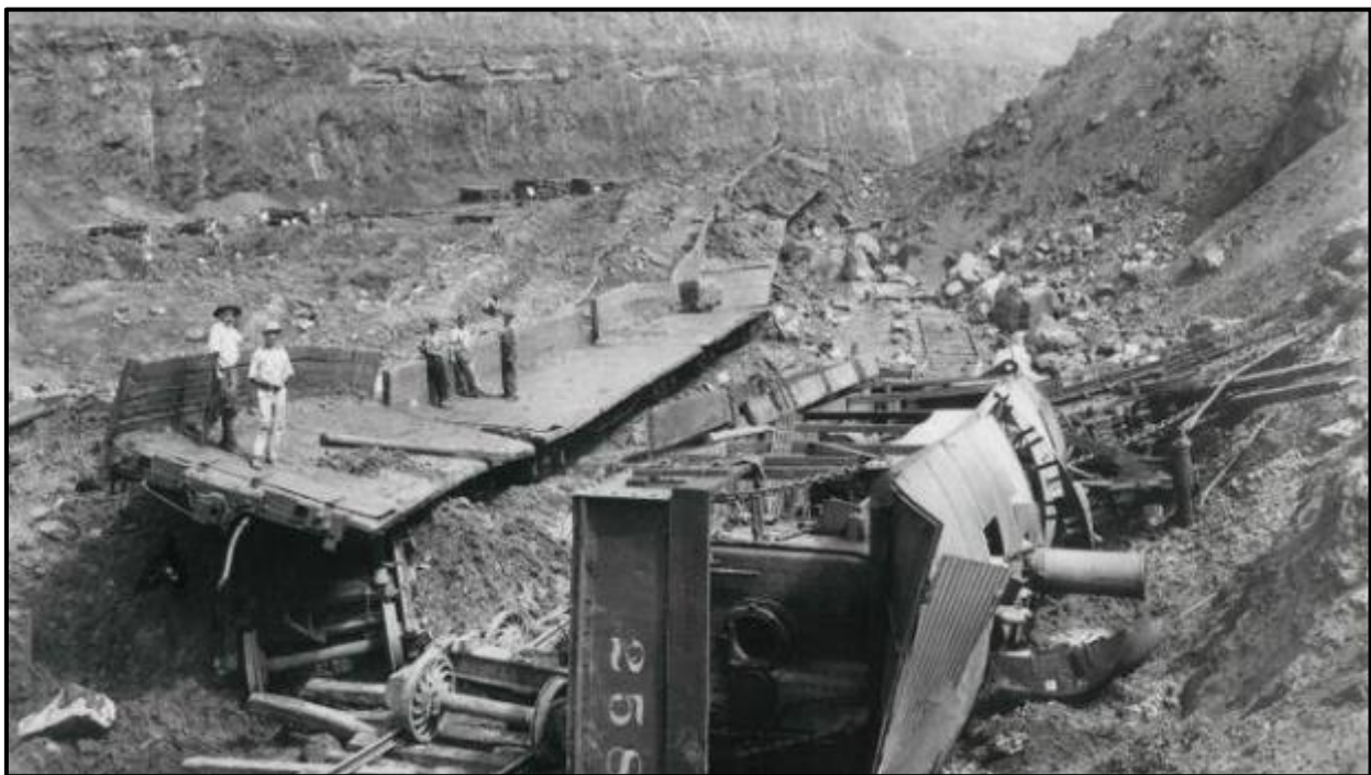
Landslide in the Panama Canal excavation
