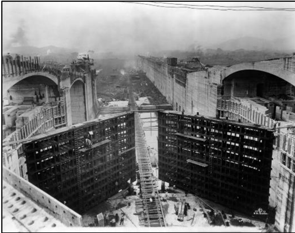
Panama Canal locks under construction http://mashable.com/2015/11/15/panama-canal-construction/#8_XsDwDN88qN
